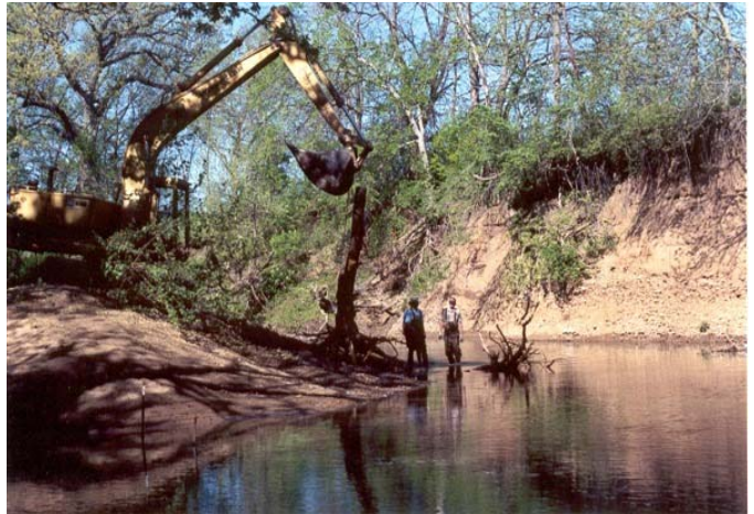
trackhoe lifting root-wad and trunk into trench
