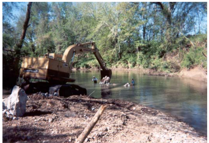
placing limestone rip-rap on lunker structures
