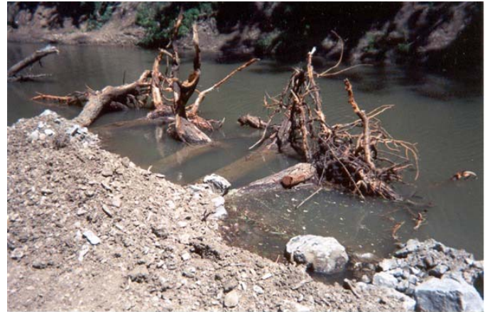
completed root-wad installation
