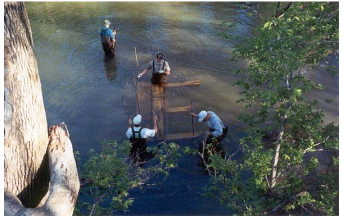
installing lunker structure
