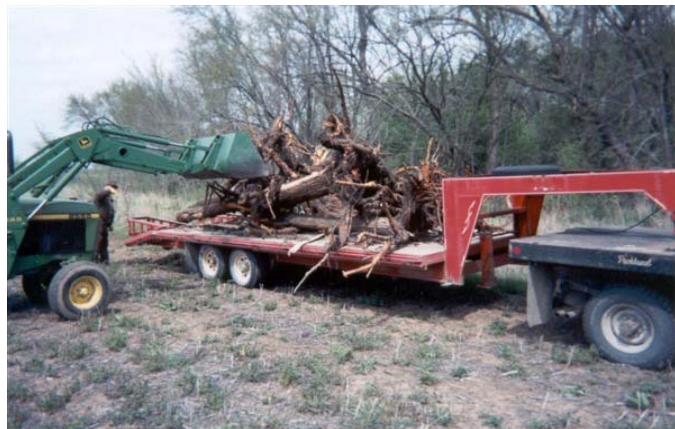
loading root-wads onto gooseneck trailer
