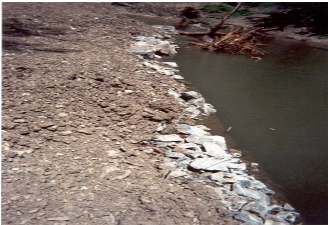
finished section of Otter Creek lunker structures
