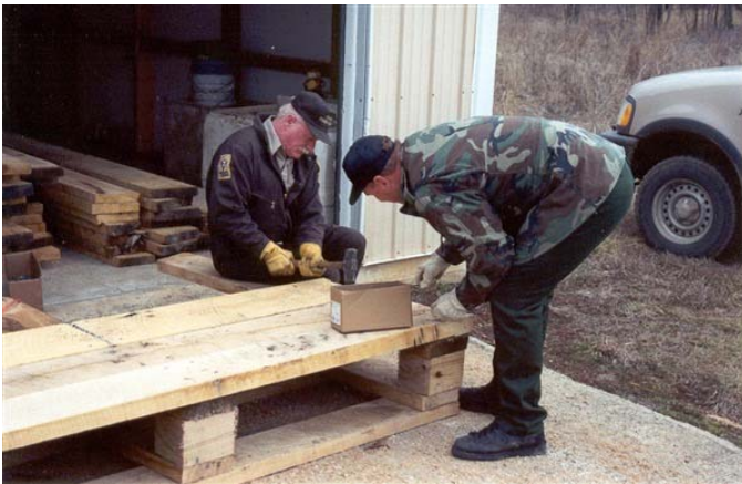
lunker structure construction
