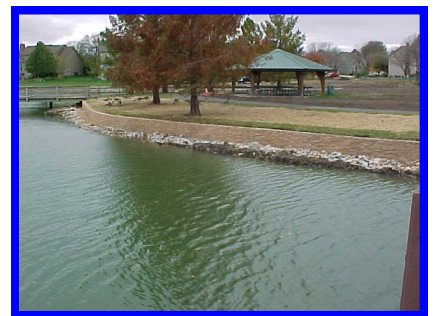
New riprap & wall at Overland Park—Kingston Lake
