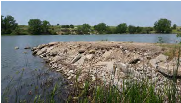
Sheridan fishing pier prior to renovation
