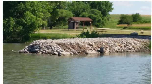
Sheridan fishing pier after renovation showing addition of new concrete
