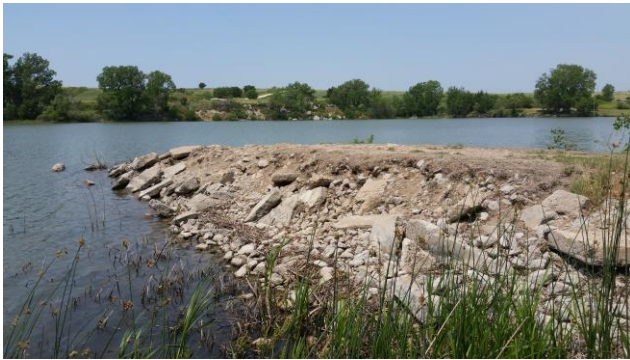
Sheridan fishing pier prior to renovation
