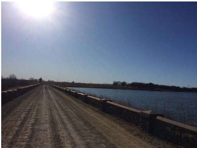
View of windgenerators across Lyon SFL Dam
